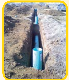
Nyloplast basin and N-12 pipe were recently installed at Los Banos High School.
